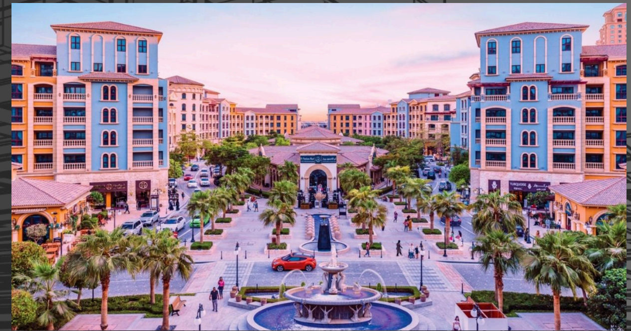
THE PEARL INTERNATIONAL Hospital QATAR
